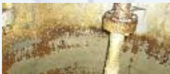
Dirty tanks with hardened products before cleaning.
