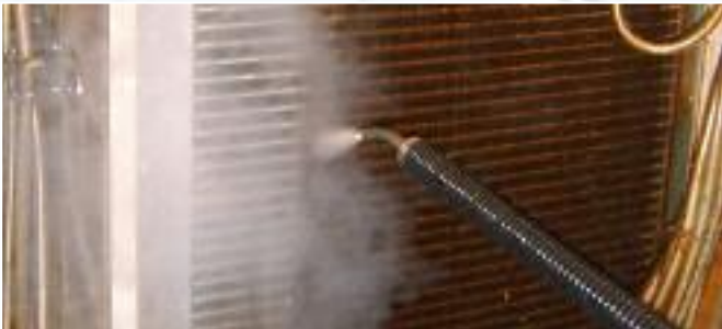
Cleaning heat exchanger.
